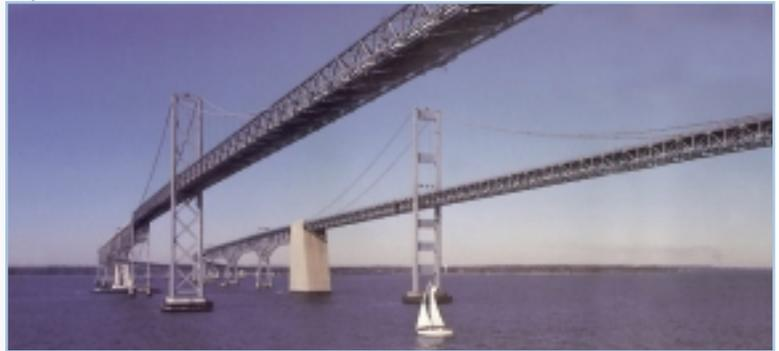
weight aggregate. Water-cement ratio was 0.40, 28-day compressive strength, 4,830 psi; and air-dry unit weight, 103# per cubic foot. In 1975, after the second parallel bridge crossing had been built, the first bridge was temporarily closed for inspection and maintenance.
