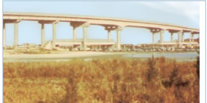
the channel opening, seemed to be the answer, except for one more problem. The US Army Corps of Engineers required that any bridge crossing the channel had to have a main span 180 feet long. This was completely unprecedented for prestressed bridge construction in Florida. Before this, the longest beam length ever used was 100 ft.
